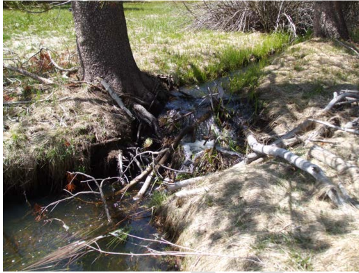
Photo 3: Looking upstream at the headcut (North Fork Angora Branch)
