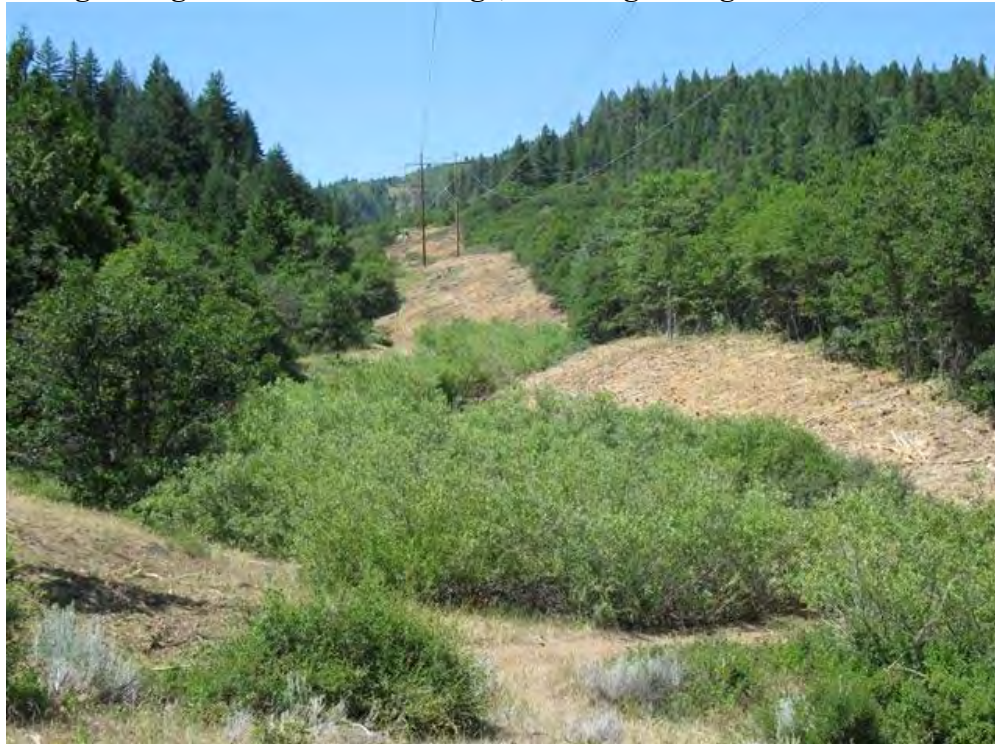
Picture 2. Additional example of post right of way clearing utilizing “Wire Zone – Border Zone” techniques on Cascade Siskiyou National Monument of Bureau of Land Management property. Low growing willow left in drainage, shorter growing oak trees left in border zone.
