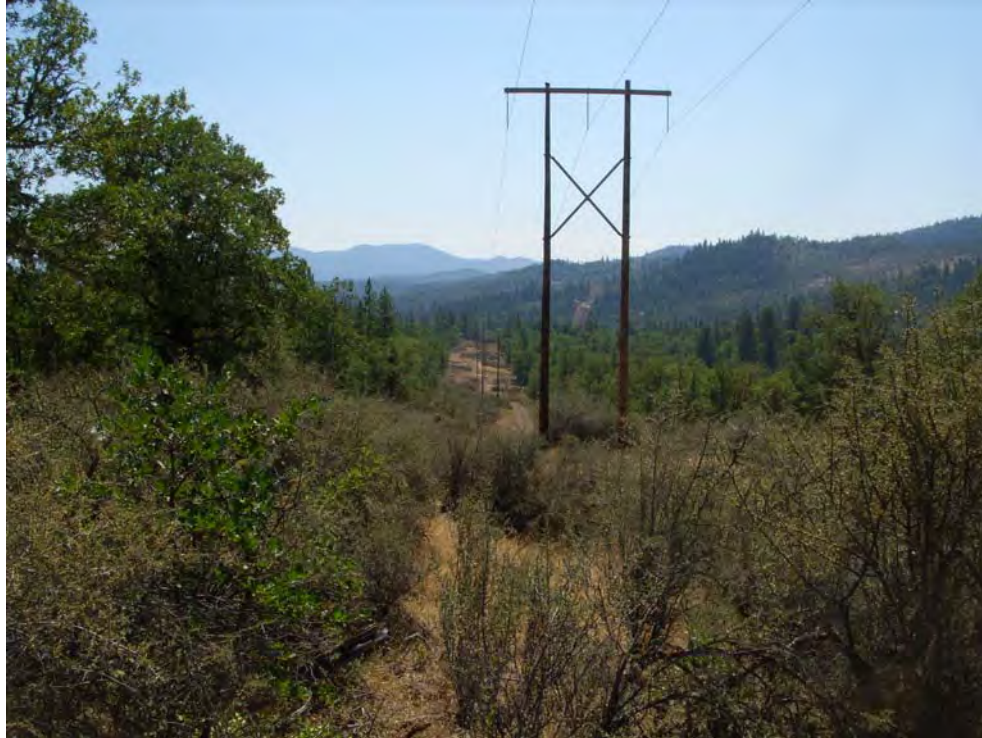
Picture 1. Example of post right of way clearing utilizing “Wire Zone – Border Zone” techniques on Cascade Siskiyou National Monument on Bureau of Land Management property. Low growing shrubs left in right of way. Shorter growing trees left in border zone.
