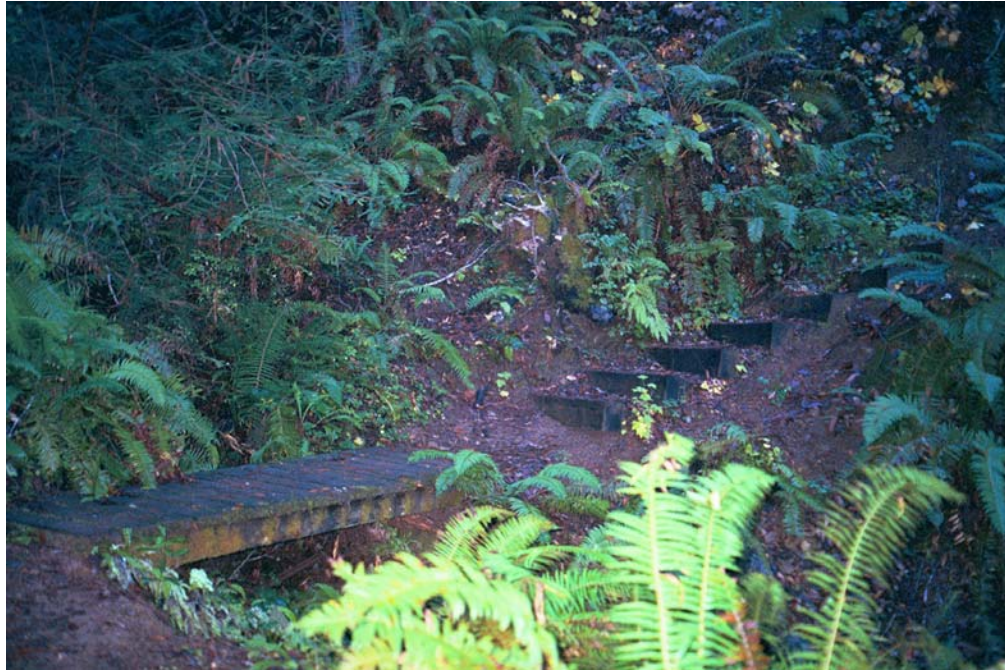
Fern Canyon Trail along Little River, Van Damme State Park. Steps down slope to puncheon bridge.
