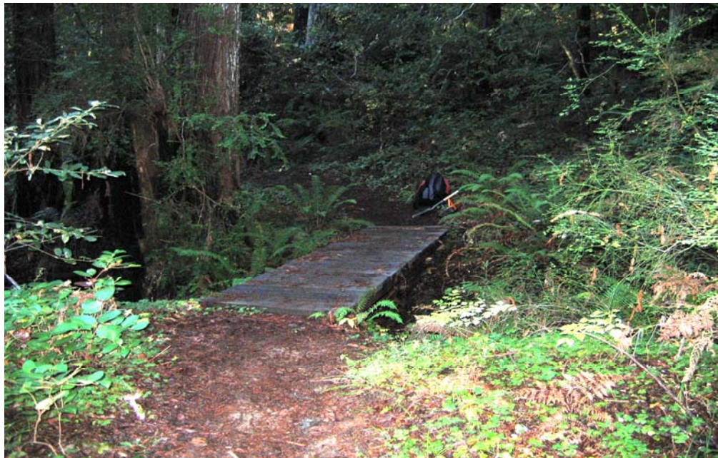
Fern Canyon Trail along Little River, Van Damme State Park. Puncheon bridge.
