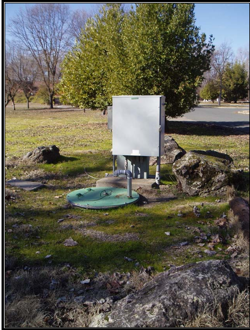
Figure 3: Existing Sewer Lift Station at Clear Lake State Park
