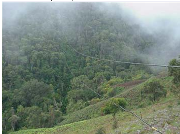
Water supply tubes in Petaquire basin, photo: Rodolfo Castillo
