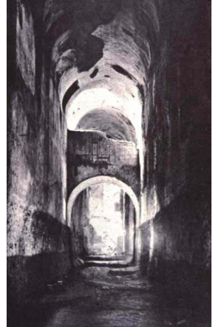
Interior hall of the Golden House
