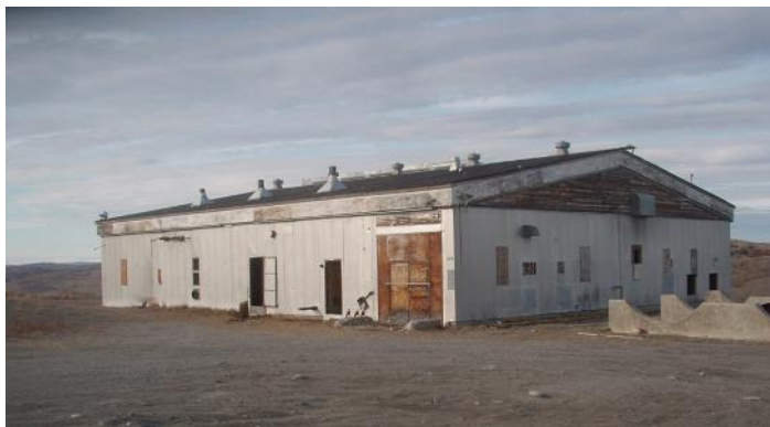
Fig. 19. The former power building near Kelly Ville
