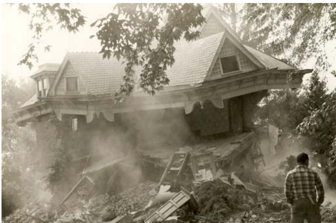
Demolition of the Forness Home on E. State (now Pool Mart)
