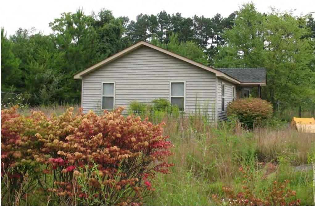
PLATE 33 Building B6 in Area B, South Facade
