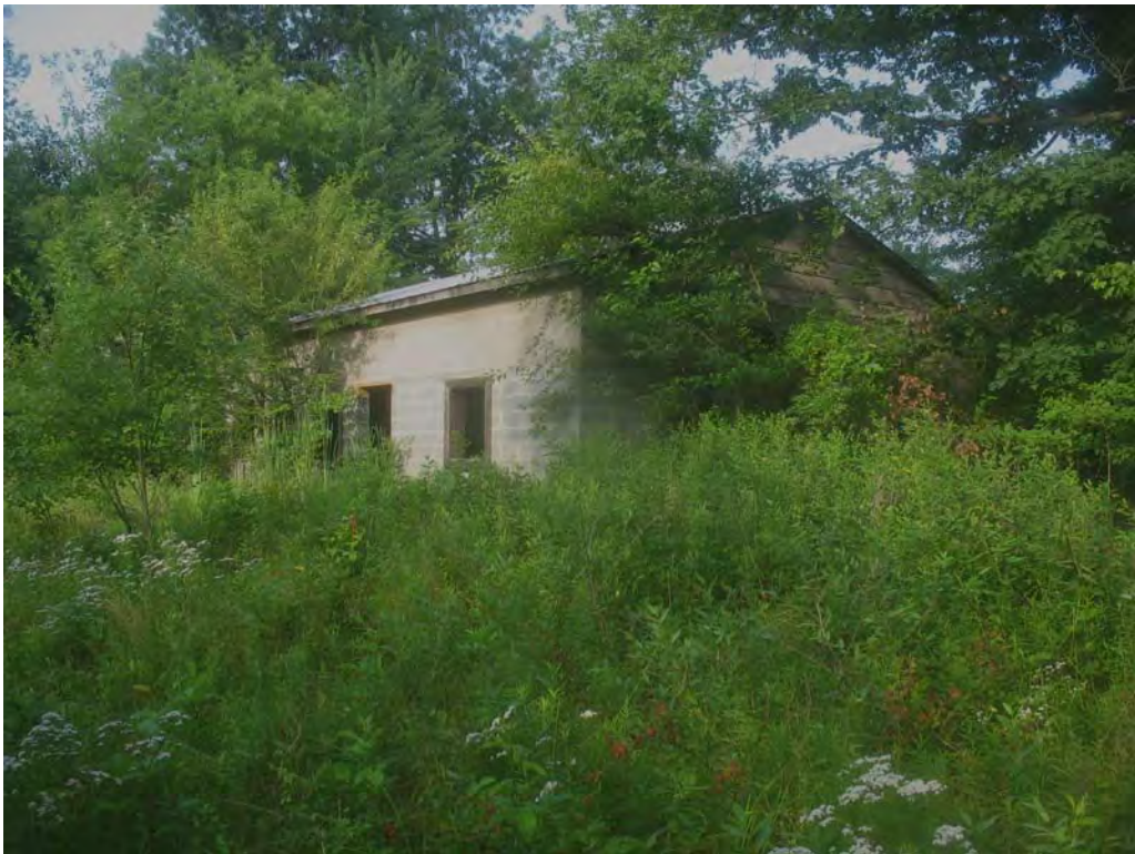
PLATE 14 Building A5 in Area A, North and East Facades
