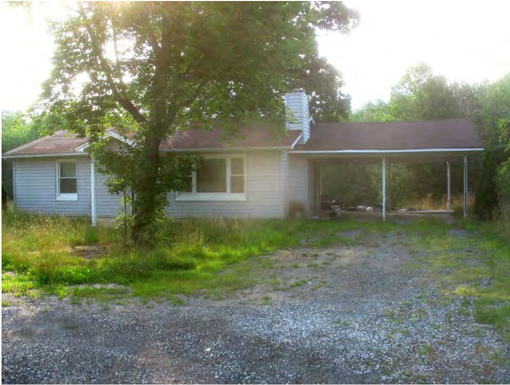
PLATE 9 Building A2 in Area A, West Facade
