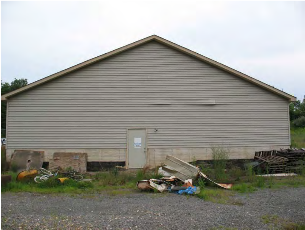
PLATE 31 Building B5 in Area B, East Facade
