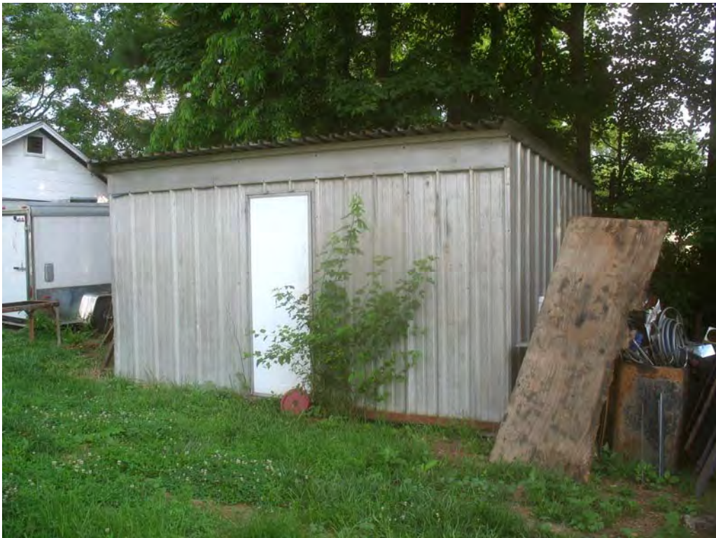
PLATE 28 Building B3 in Area B, East Façade
