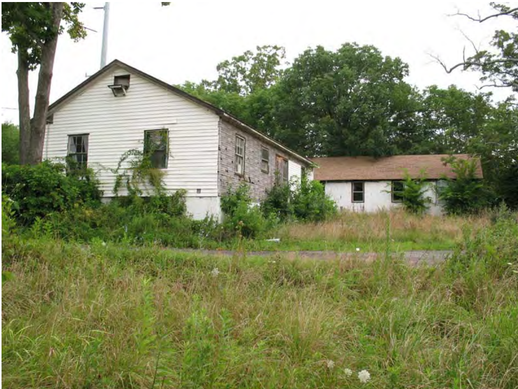
PLATE 6 Building A1 (DHR 076-5181) in Area A, South Façade
