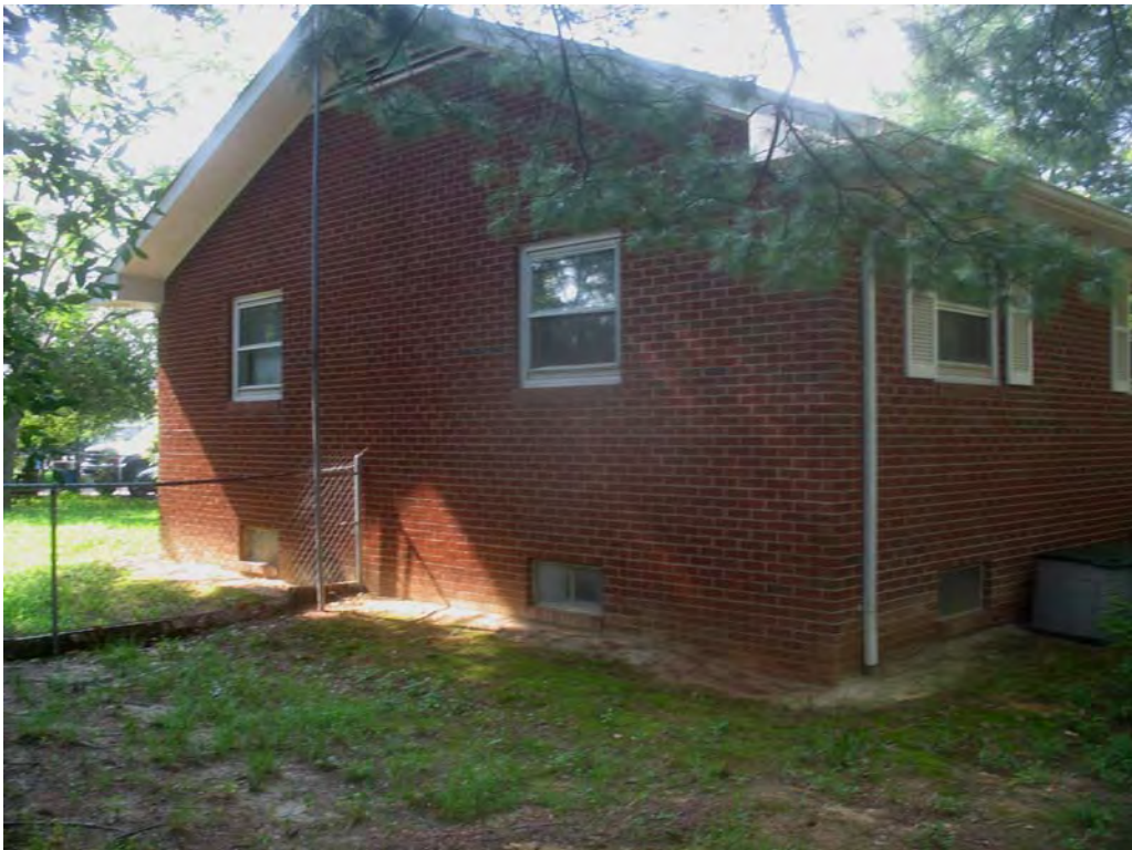
PLATE 26 Building B1 in Area A, North Façade
