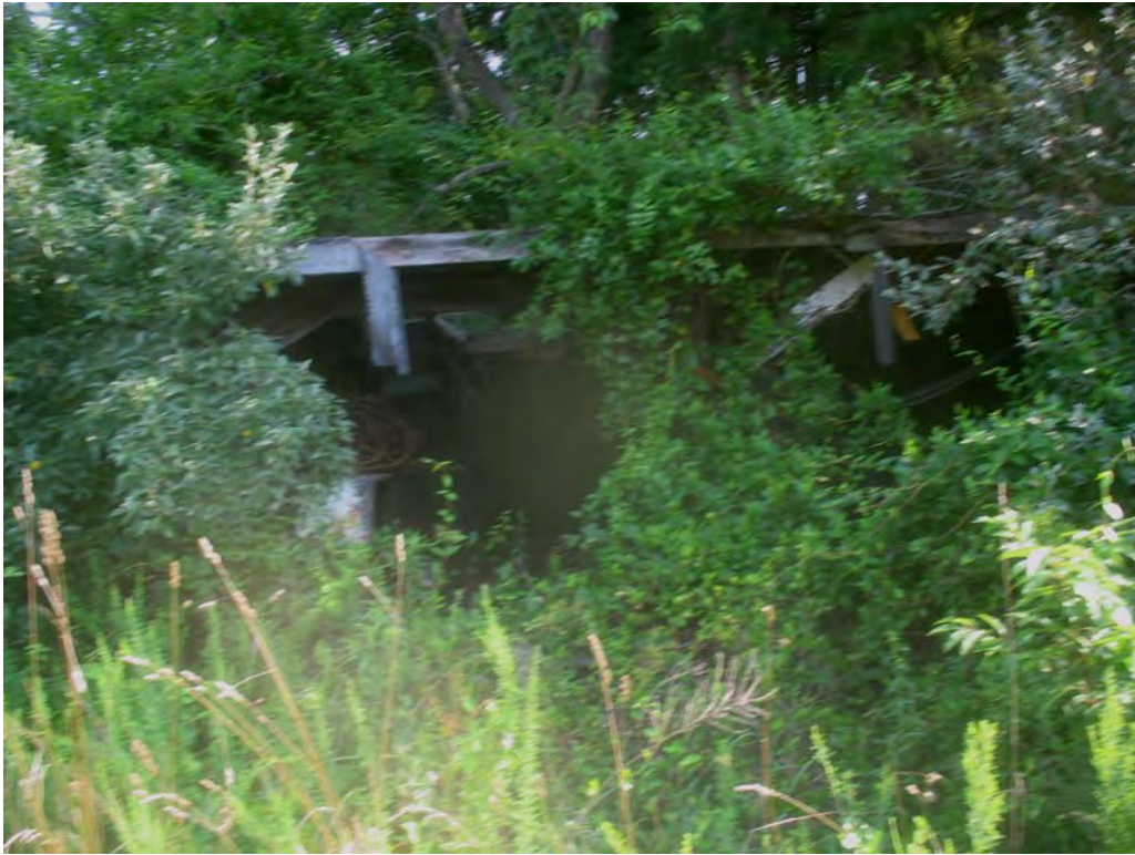
PLATE 29 Building B4 in Area B, View to North
