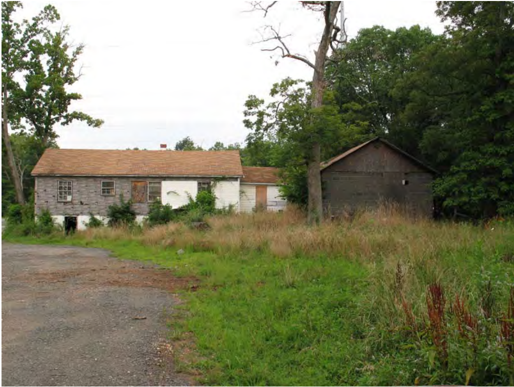
PLATE 7 Building A1 (DHR 076-5181) in Area A, East Facade
