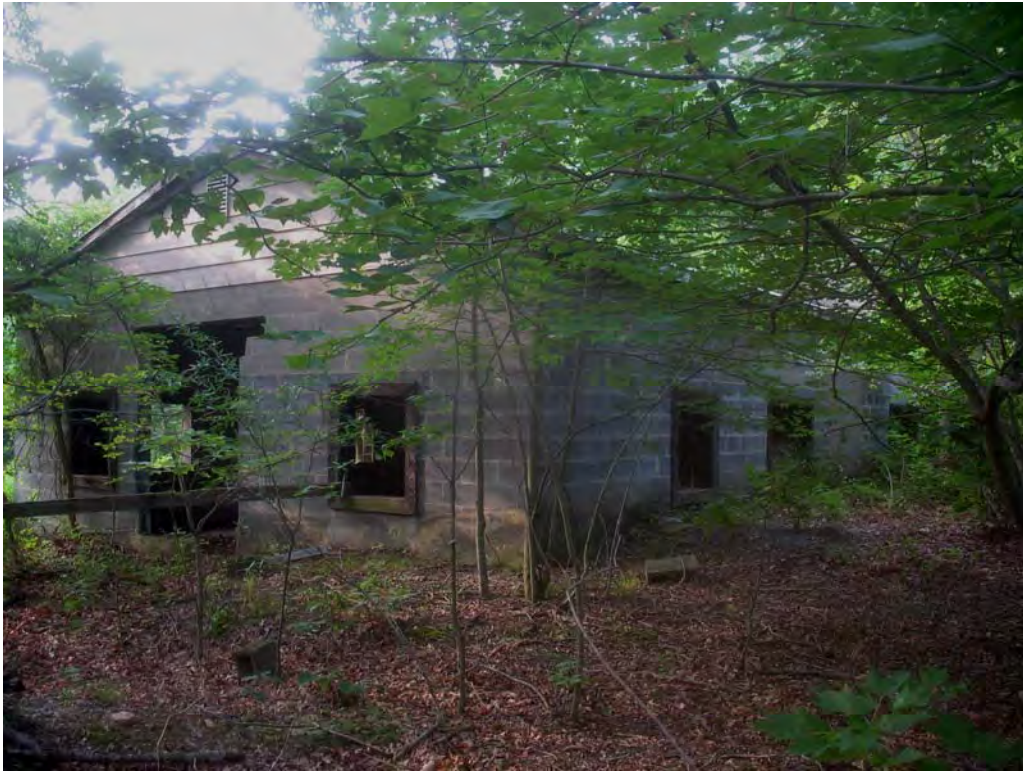
PLATE 13 Building A5 in Area A, North and West Facades
