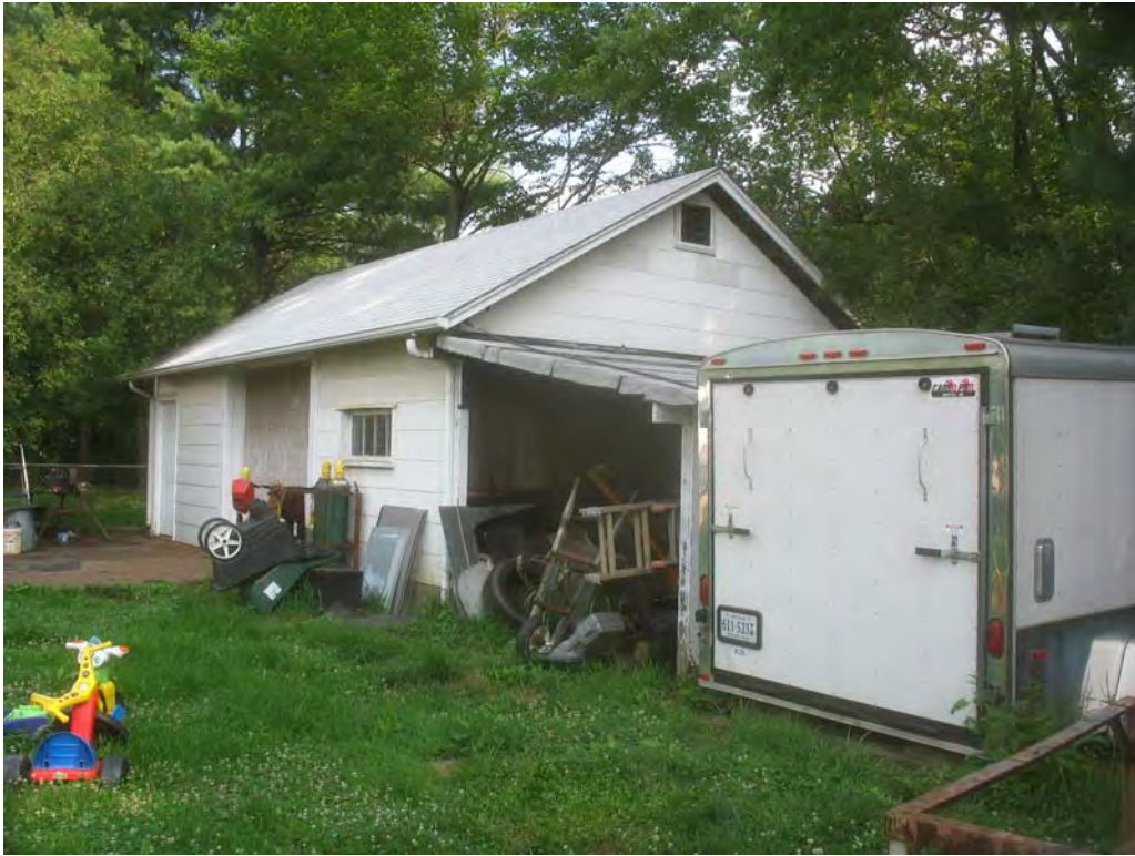
PLATE 27 Building B2 in Area B, South and East Facades
