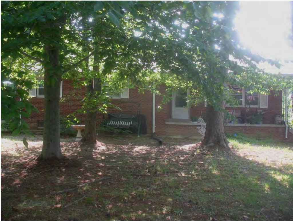
PLATE 23 Building B1 in Area B, West Façade
