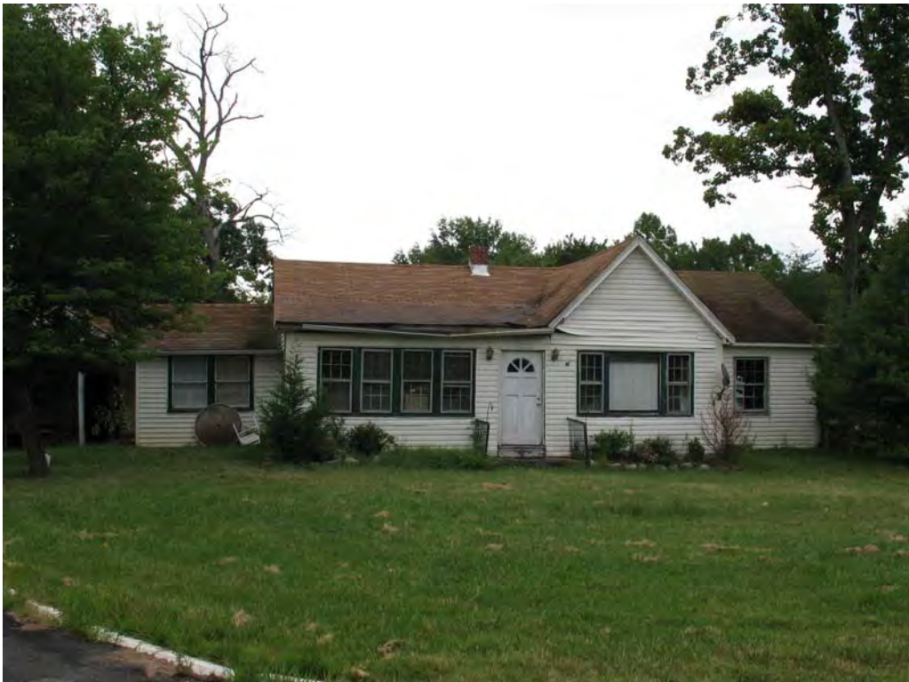
PLATE 4 Building A1 (DHR 076-5181) in Area A, West Façade
