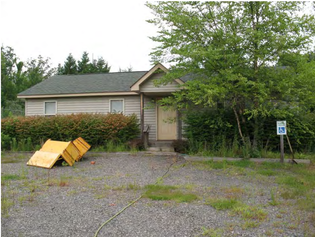
PLATE 32 Building B6 in Area B, East Façade
