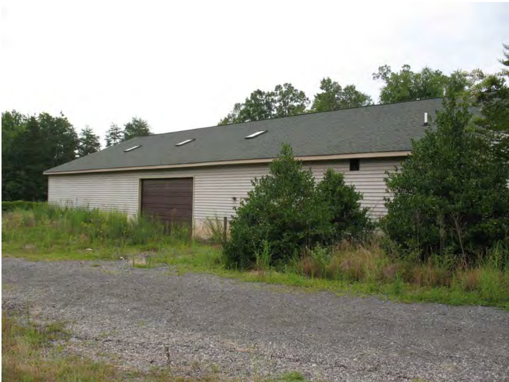
PLATE 30 Building B5 in Area B, North Facade
