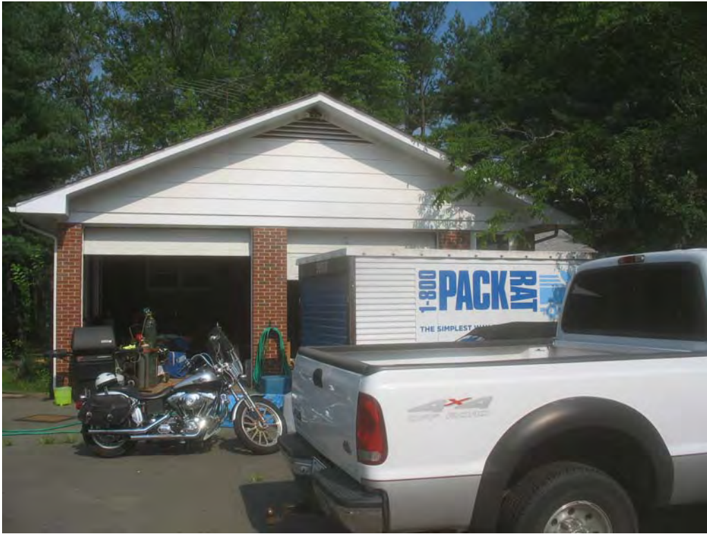
PLATE 25 Building B1 in Area B, East Façade
