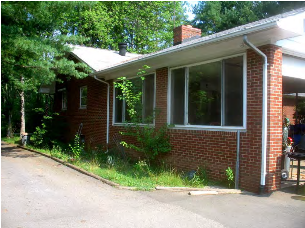
PLATE 24 Building B1 in Area B, South Façade
