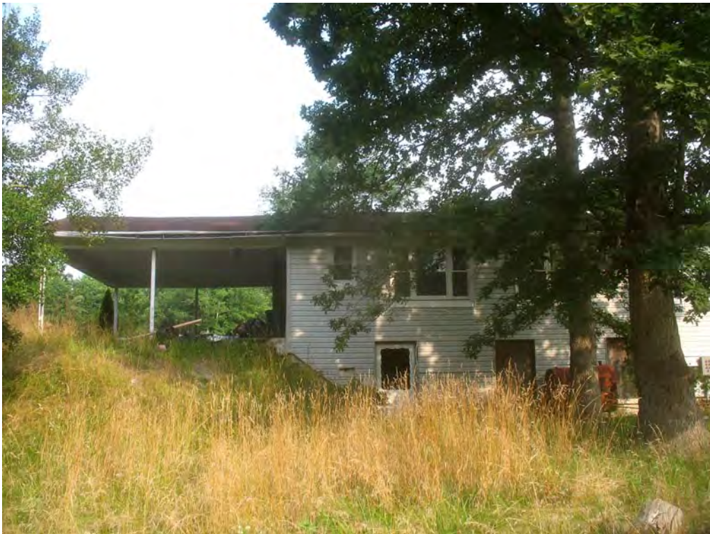
PLATE 10 Building A2 in Area A, East Façade
