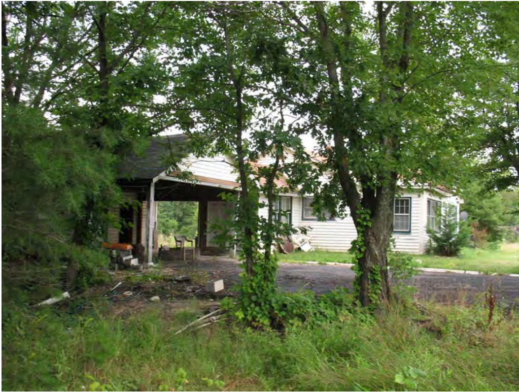
PLATE 5 Building A1 (DHR 076-5181) in Area A, North Façade
