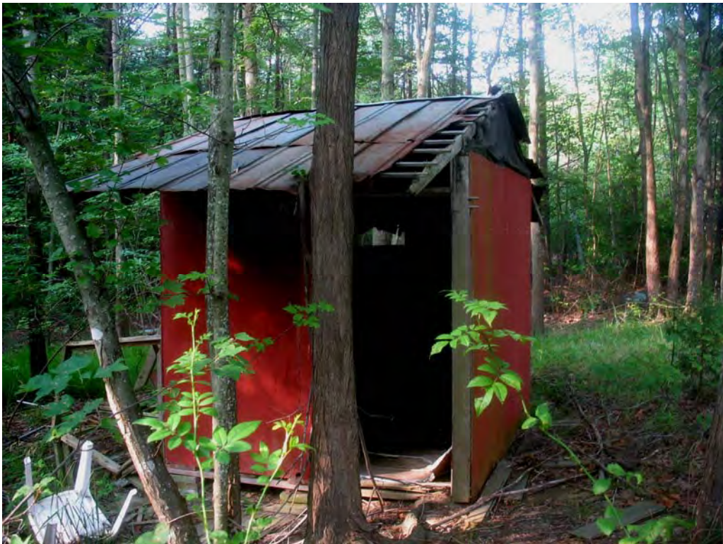
PLATE 12 Building A4 in Area A, View to Southeast
