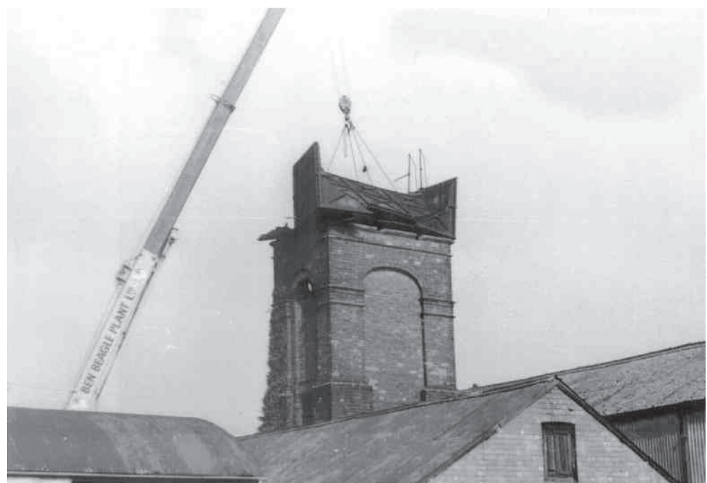
The water tower and storage tank being dismantled.
