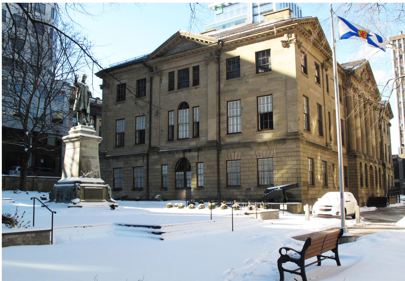
Exterior shots of Province House from 2007 (above) and 2019 (below)
