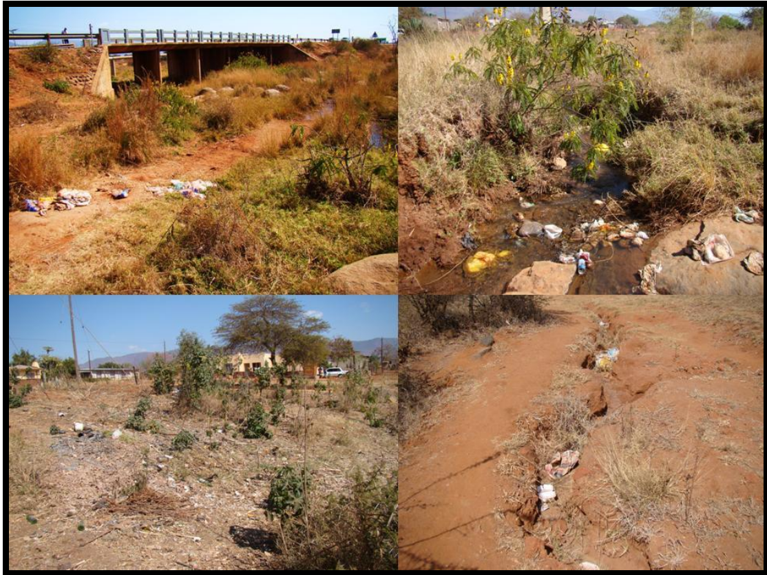
Figure12. A conglomerate of photographs displaying the current impacts observed at the Rooisloot bridge crossing; (A) : The area around the current bridge is heavily degraded due to high levels of human disturbances within the active channel as well as macro-channel banks of the Rooisloot as well as adjacent riparian zone has resulted in habitat destruction and degradation as well as deterioration of water quality; (B & C) : Evidence of vegetation clearance and wood harvesting within the riparian zone as well as alien vegetation invasion, extensive littering and illegal dumping activities within the active channel as well as macro-channel banks; (D) : Erosion channels from surface runoff from the road entering through eroded channels directly into the Rooisloot; resulting in increased levels of siltation and sedimentation within the river.
