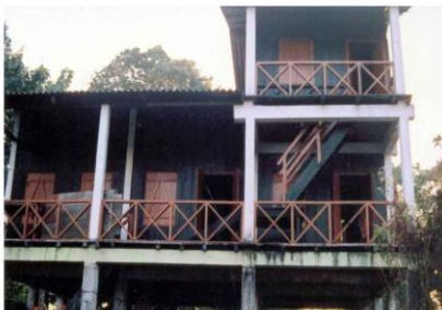
Plate 12 : Restoration of forest camp
