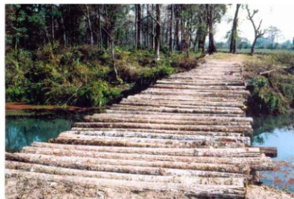
Plate 16: Restoration of boundary bridge
