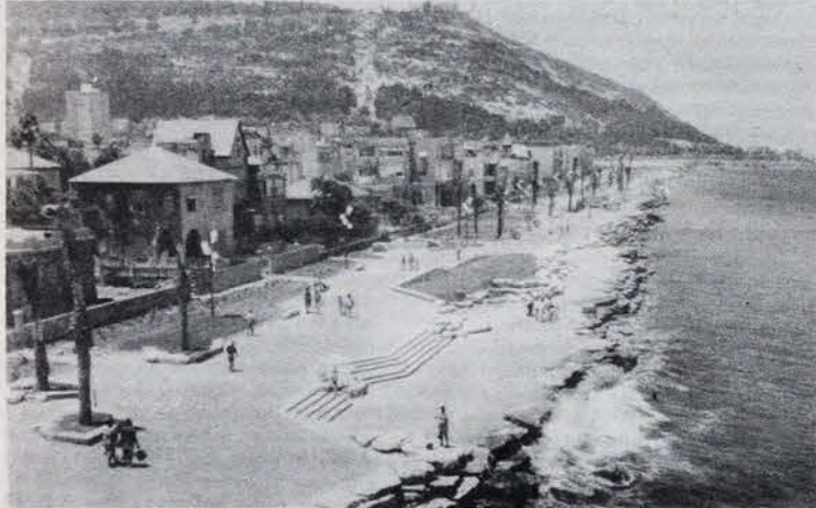
The newly completed sea-front at Bat-Galim Promenade in Haifa.
