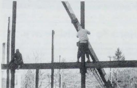
Construction begins on the Solomon Schechter School in Providence.
