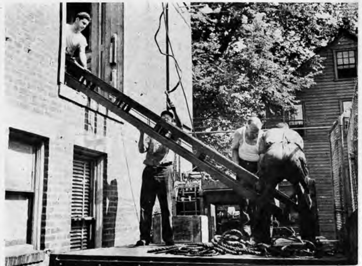
The camera cradle or bed is hoisted and lifted to the loading truck. Note its extreme length—the far end of the machinery is still inside the plant.
