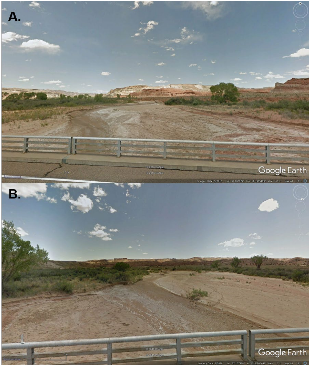
Figure 1.4-1. Upstream (A) and downstream (B) views of the Paria River at the Proposed Project U.S. Highway 89 crossing in May 2018 (Source: GoogleEarth 2018, as modified by Commission staff).
