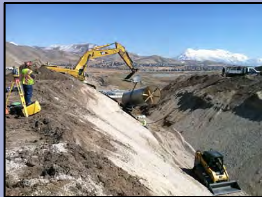
Provo Reservoir Canal Enclosure Project Source: Jordan Valley Water Conservancy District
