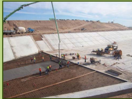
All-American Canal lining in progress
