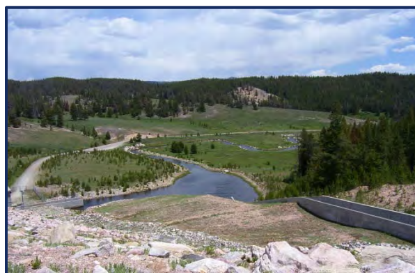
Hog Park Reservoir Outlet, web camera image from October 29, 2014
