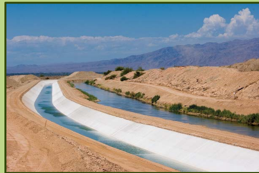
Water begins to flow through the new canal adjacent to the original earthen structure
