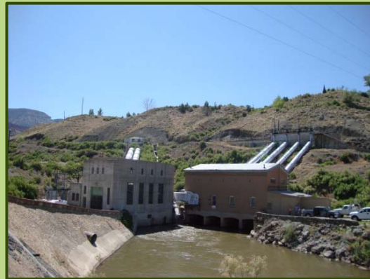
Orchard Mesa Pumping Plant
