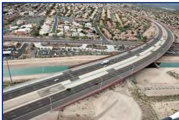
Central Arizona Project aqueduct delivers Colorado River water to Pima, Pina, and Maricopa Counties Source: Central Arizona Project
