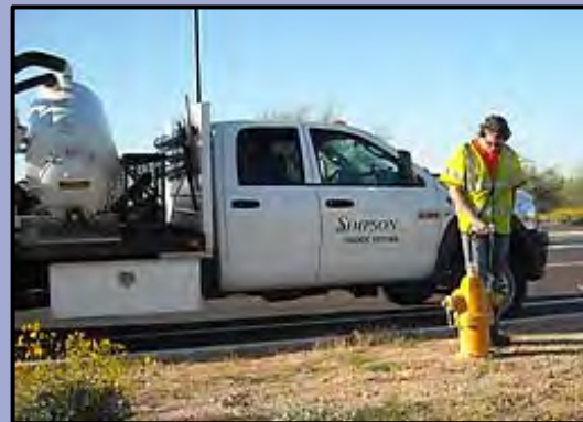
Using a Correlator Microprocessor Unit to Determine Leak Location
