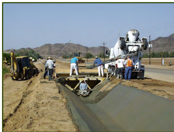
Dome Canal lining
