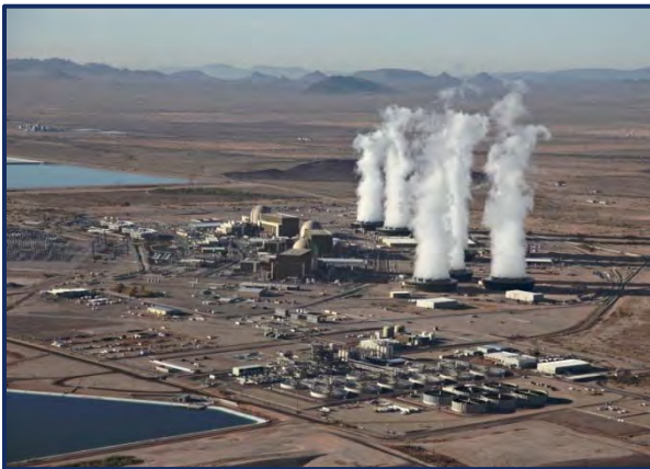
Palo Verde Nuclear Generating Station Source: Arizona Public Service Company
