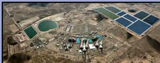
Palo Verde Nuclear Generating Station Source: Arizona Public Service Company
