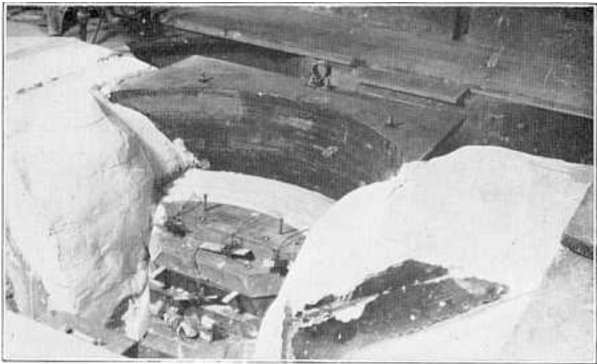
FIGURE 39—MODEL POURED TO ELEVATION 950
