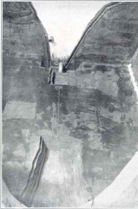
FIGURE 186—MODEL AND CANYON BUILT TO ELEVATION 595 Rods in Place for Measuring Downstream Movement of Upstream Face and Center Line
