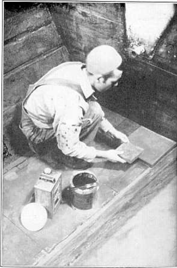
FIGURE 181—CONSTRUCTING THE SUPPLEMENTAL BASE
