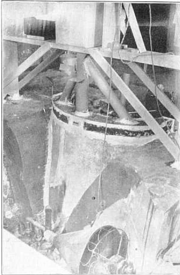
FIGURE 129—MODEL READY FOR TEMPERATURE TEST
