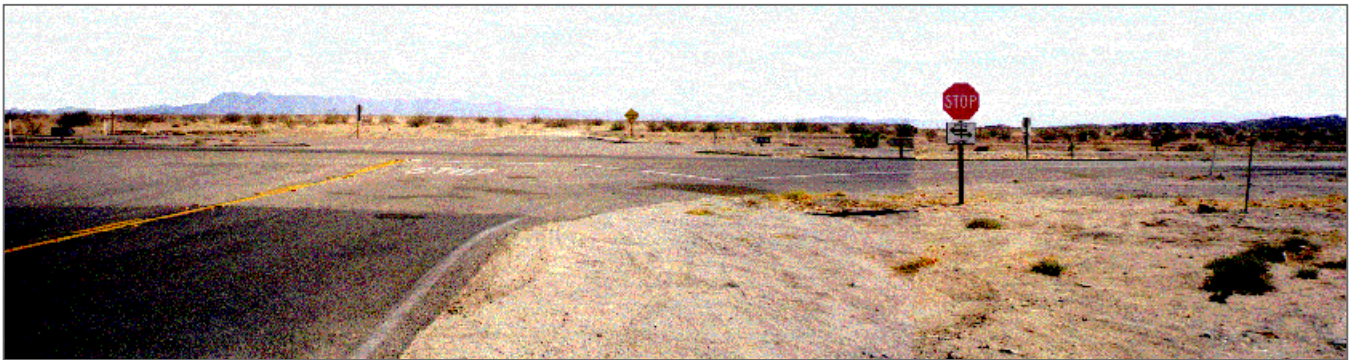
2 State Route 86, entrance to Salton Sea Test Base, location of road crossing for haul road. Looking West.
