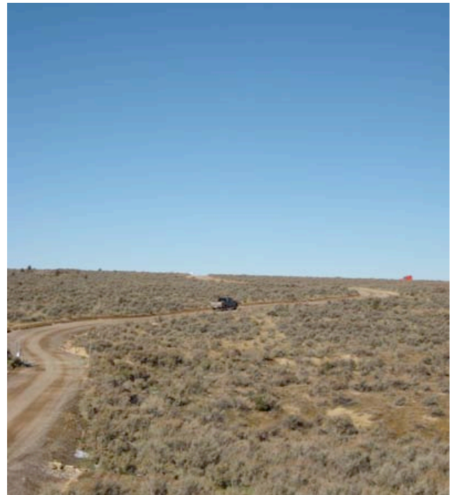
A dirt road cuts through the sagebrush landscape near the Chevron RD&D lease site, providing access to oil and gas operations in the area. Roads can have a major impact on ecosystems, providing an entry point for invasive species and disrupting wildlife movements. Credit: Jason L. Hanson (Oct 2007)
