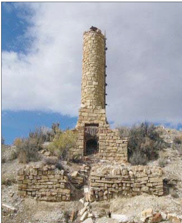
When the first oil shale boom went bust in the 1920s, companies abandoned Shale Country as quickly as they had appeared, leaving the ruins of retorts such as this one on Willow Creek southwest of Vernal, Utah, as monuments to their failed efforts. Credit: National Energy Technology Laboratory
