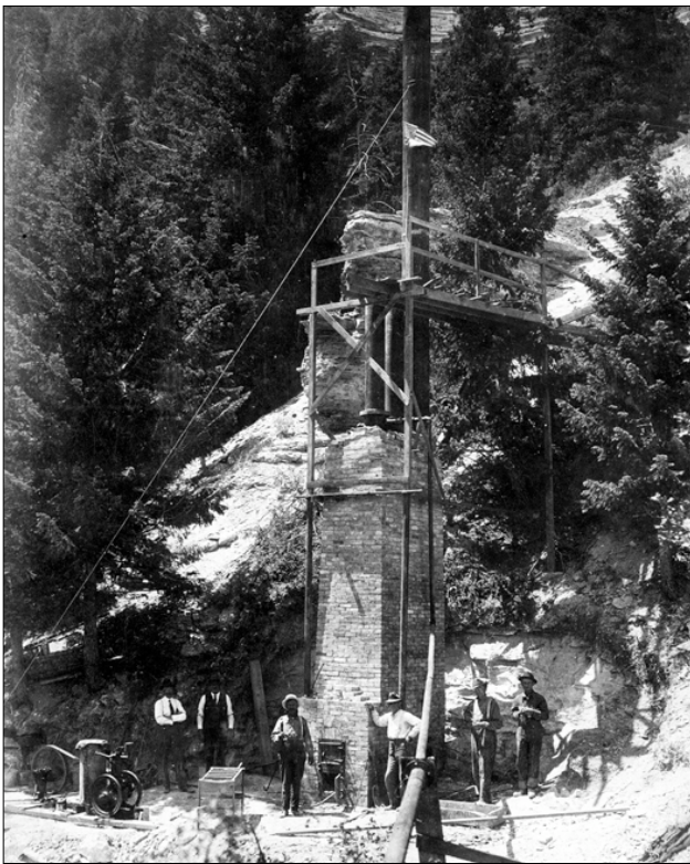
The first oil shale retort in Colorado, shown here in a photograph printed in National Geographic in 1918, was built by the Oil Shale Mining Company on Dry Fork west of De Beque, Garfield County, Colorado. Designed from illustrations found in the Encyclopedia Britannica entry on the Scottish oil shale industry, the retort heated crushed shale to extract oil. Credit: US Geological Survey
