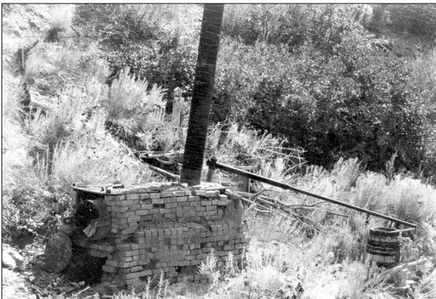
The old Mormon Retort near Levan, Juab County, Utah, photographed in 1916. Built by Mormon pioneers roughly 60 years earlier, it was the first known oil shale operation in the Rocky Mountain West, extracting as much as a barrel of oil a day from the surrounding rocks for use in dressing leather harnesses, lubricating wagon wheel axles, and lighting lamps. Credit: US Geological Survey
