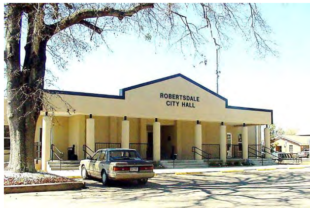
Photograph 9.1: Robertsdale City Hall
