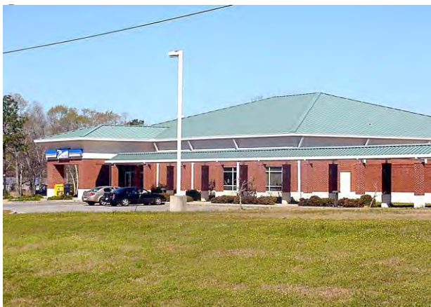
Photograph 9.7: Robertsdale Post Office
