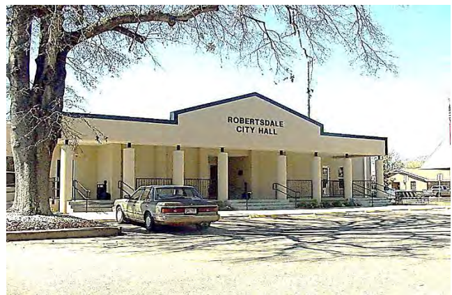
Photograph 1.3: Robertsdale City Hall
