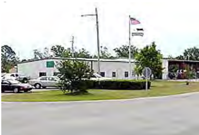
Photograph 9.2: Department of Public Works
