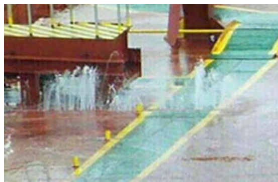
Cracks on the Stellar Queen's deck.
