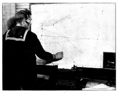
PLOTTING A SHIP'S POSITION The compass bearings of a given ship, reported to the central station in New York by several radio compass stations, are indicated by lines drawn from the receiving stations on a map. The ship's position is the point at which the lines cross
