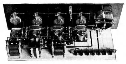
FIG. 2 The Interior of Mr. Zieger's set. Note the rear connections, the neat wiring, and the placing of the transformers
