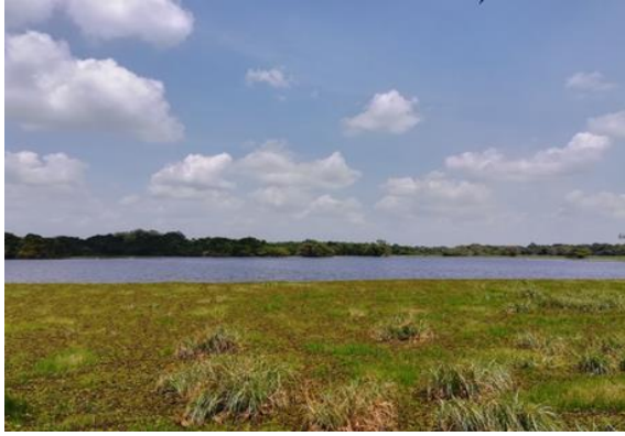
Plate 2.6. Initial stages of weed and bush encroachments into the tank can be seen in some tanks and regular maintenance needs to be scheduled
