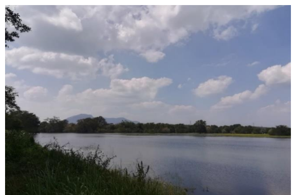
Plate 2.9. Considerable number of tanks are well functioning and properly maintained and can be considered as best models
