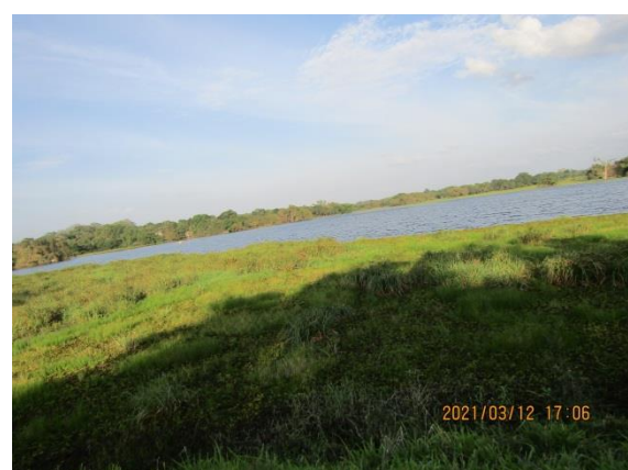
Plate 3.2.11. Severe aquatic weed invasion in bund side-Sembukulama tank
