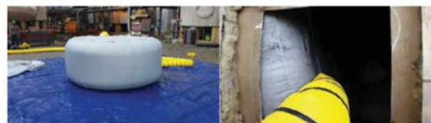
Figure 10—Duct balloons used for isolation
