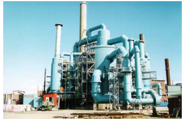
Figure 2—Chemetics five-pass converter with two internal heat exchangers
