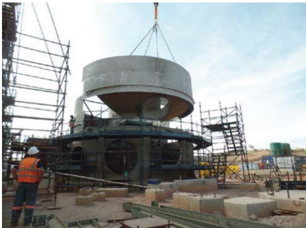
Figure 8—Converter modules assembly on site
