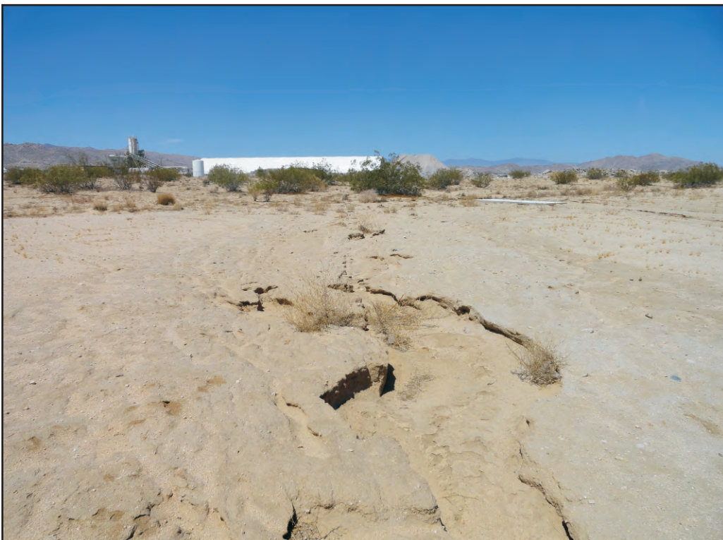
Photograph 4 - Airport property, APN 0607-231-09, view to the southwest. View of minor erosion features associated with the southern portion of the earthen runway.
