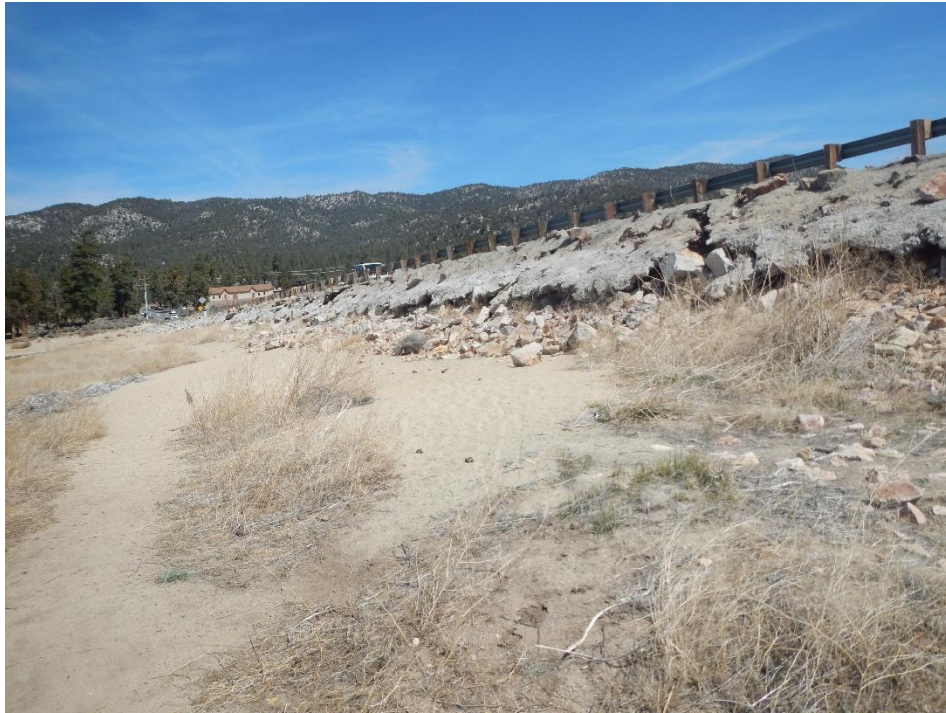
Photo 3: Big Bear Lake bank scour along the western border of Stanfield Cutoff, looking northeast.
