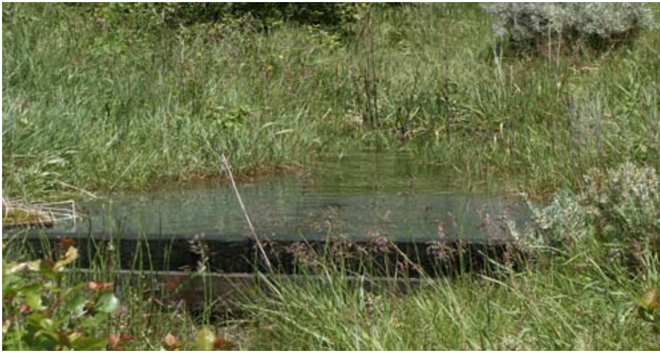
Looking upstream toward the dam
