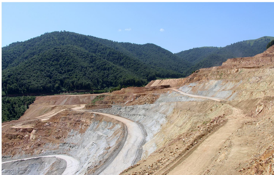
Fig. 2. The deforested area A of the surface mine surface (photo. O. Majzlan, 20.3.2016).
