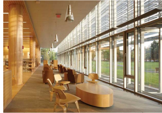
Figure 4. View towards double skin façade on the first floor.
