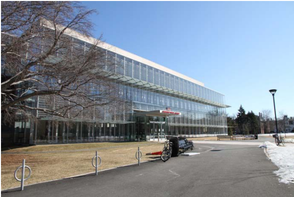
Figure 2. New addition to the historic Cambridge library.
