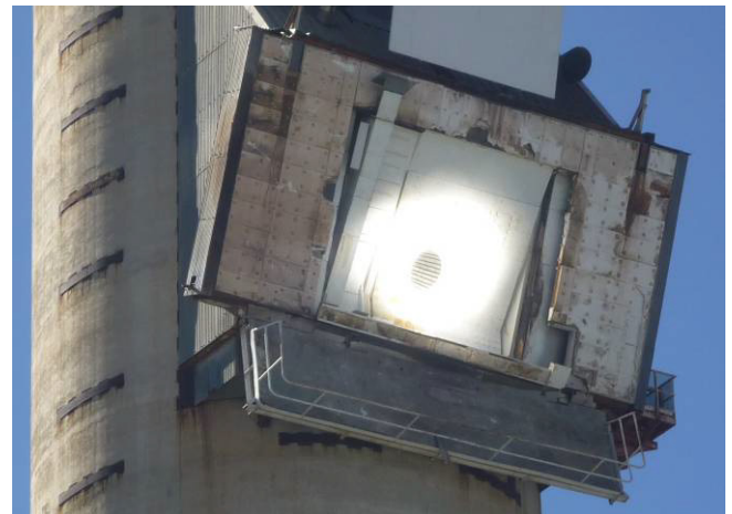
Figure 5.10 Operation of the Solhyco prototype system in the CESA-1 tower
