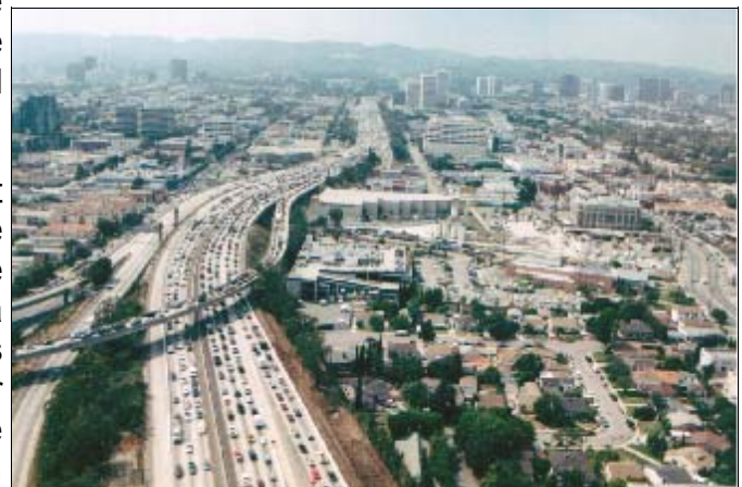
The Los Angeles 405 Freeway as seen from the "Spirit of Freedom".
