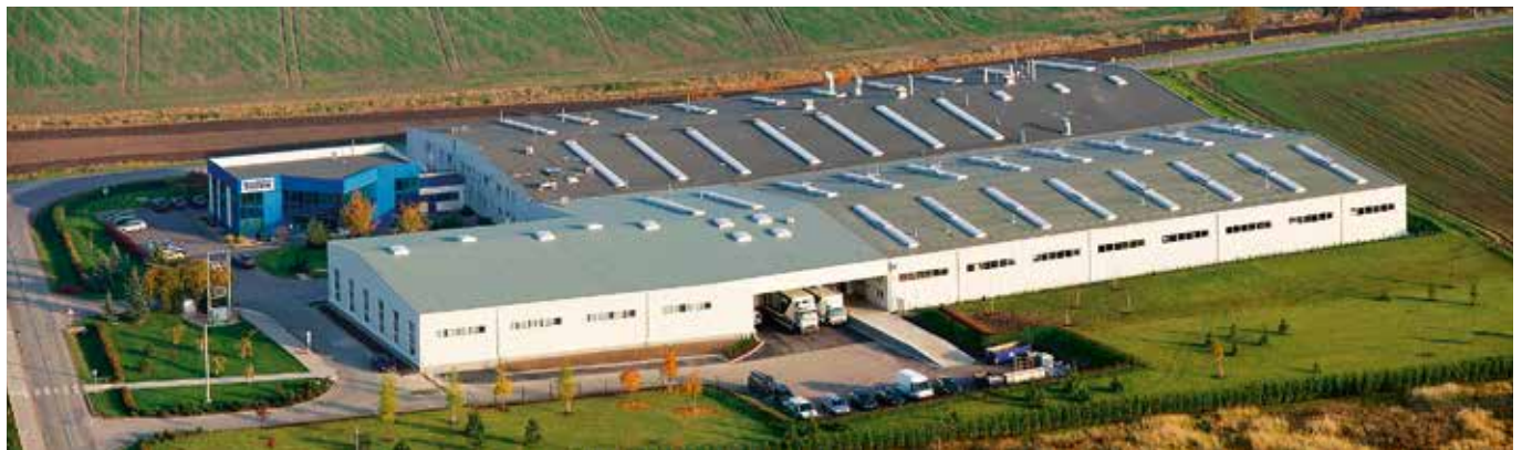
Year 2011 - extension of the third hall - new warehouse and logistics
