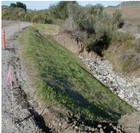
Just after completion
