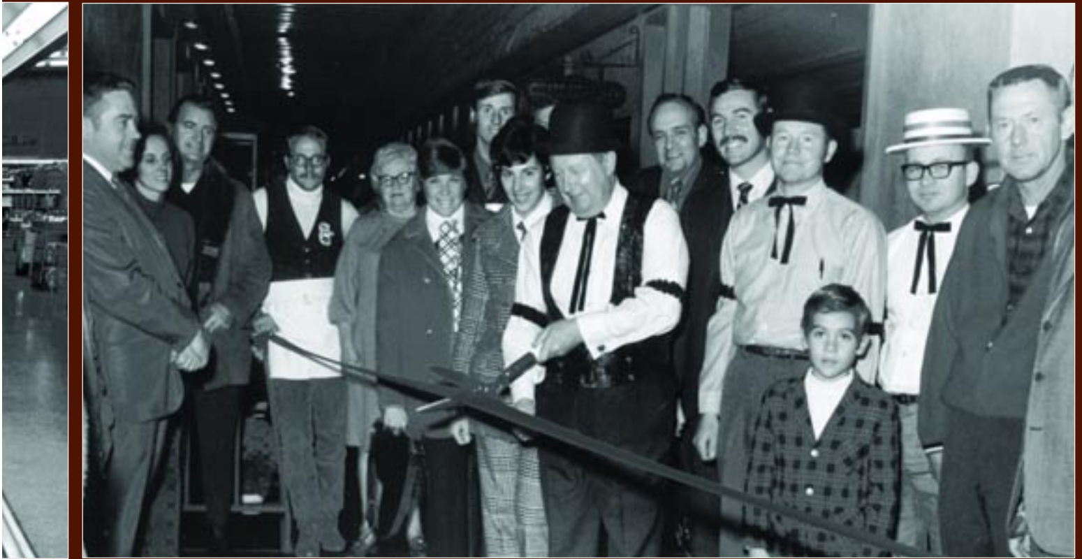
1969: Atkinsons' Market's founder, Charles "Chuck" Atkinson, cuts the ribbon and officially opens Giacobbli Square, the location of their new store. To the right of Chuck is George Hellyer, Don's brother-in-law, who built the building. To the right of George are Chuck's sons, Don—the store's manager, and Stan—the meat department manager and assistant store manager, who continued their father's vision into the next century. Also pictured are Chuck's wife, Flossie, (back center with glasses) and Don's wife, Judy (to the left of Chuck), who designed the interior of the new store.
