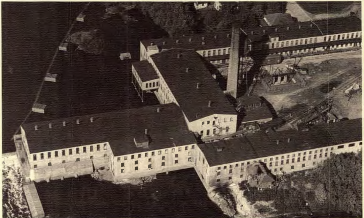
An early aerial view of the Whiting Plover Paper Company. Raw materials entered at the lower portion of the "U" shaped building
