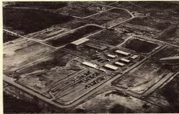
An early airview of construction of the Ashdown mill. The buildings with the white roofs are buildings erected first to be used as headquarters and shops for the contractor. The warehouse to the rear was built first to provide a place to store incoming parts.
