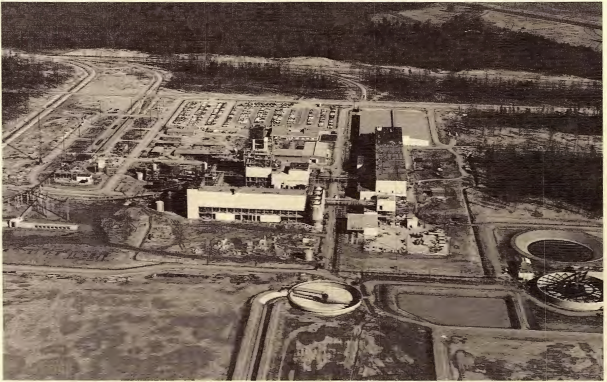
Illustrated is the Ashdown mill after completion of phase one.
