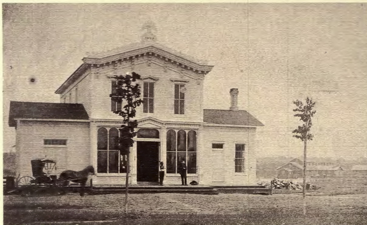
John Edwards, Jr. built this office building in 1872 to serve the administrative needs of his lumbering operation. In later years
