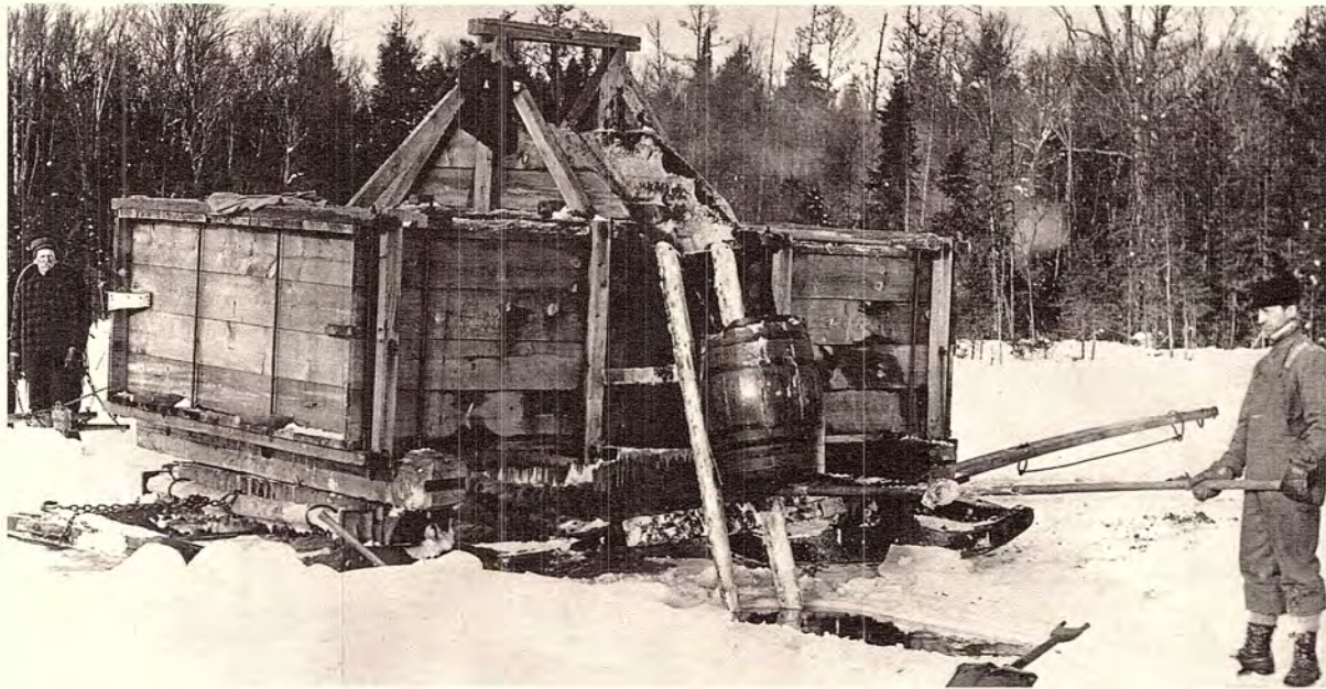
The coldest job in a lumber camp was to go out at night on the icing sleigh. Here, such a sleigh is being loaded with water in preparation for icing the roads.
