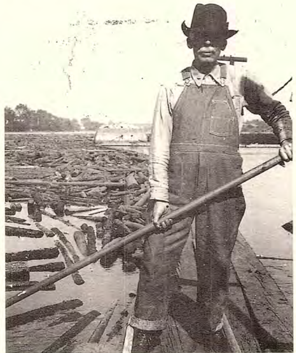
A lumber mill employee with his pike pole works the boom above the dam at Port Edwards.
