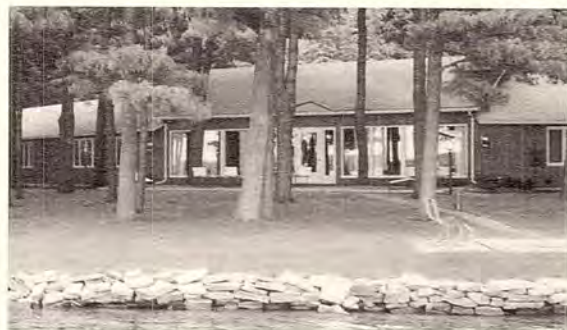
When the Port Edwards hotel was no longer available for hosting visiting customers, Nekoosa Papers Inc. built this guest house on the north shore of Nepco Lake. It was named Nekoosa Lodge and accommodated 12 people for overnight visits.
