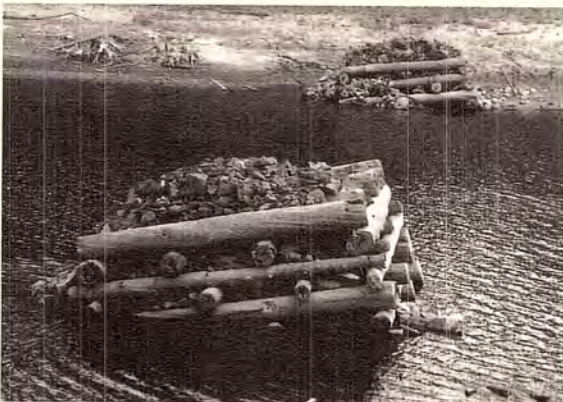
Cribs of rock are still quite plentiful under the surface of the river. These two are just off of the end of Market Street.
