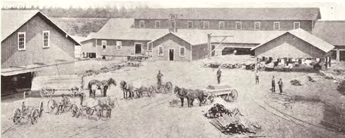
The John Edwards Lumber Company in the late 1870s. The railroad tracks lead only as far as the lumber storage piles.
