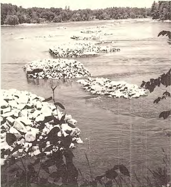
Port Edwards received its name because it was a log and lumber port. Here are some of the rock cribs to which booms were attached for holding logs and lumber rafts in this river port.
