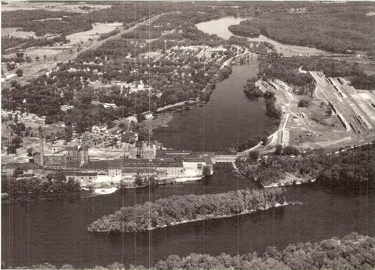
Air view of the Port Edwards mill, island log yard, and part of the village in the early 1940s.
