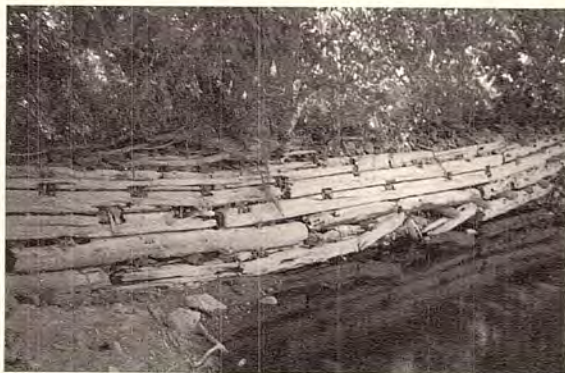
The west bank of the river still has a log diversion wall opposite the Alexander House. This was to divert logs to the channel of the stream.
