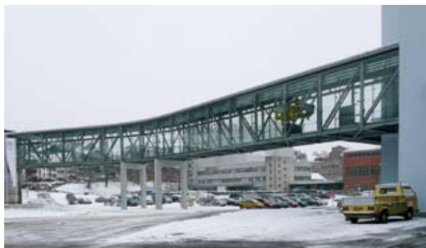
Steeltec: Logistics bridge for wire rod delivery
