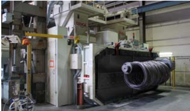
Ugitech: New descaling plant
