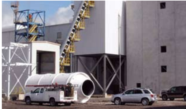
A. Finkl & Sons: Reconstruction of the steel plant
