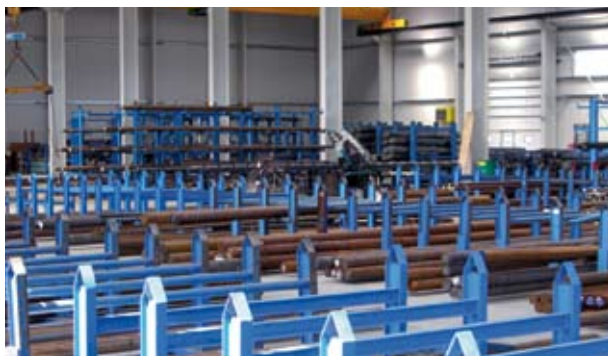
SCHMOLZ + BICKENBACH Distribution Europe: New warehouse in Slovakia
