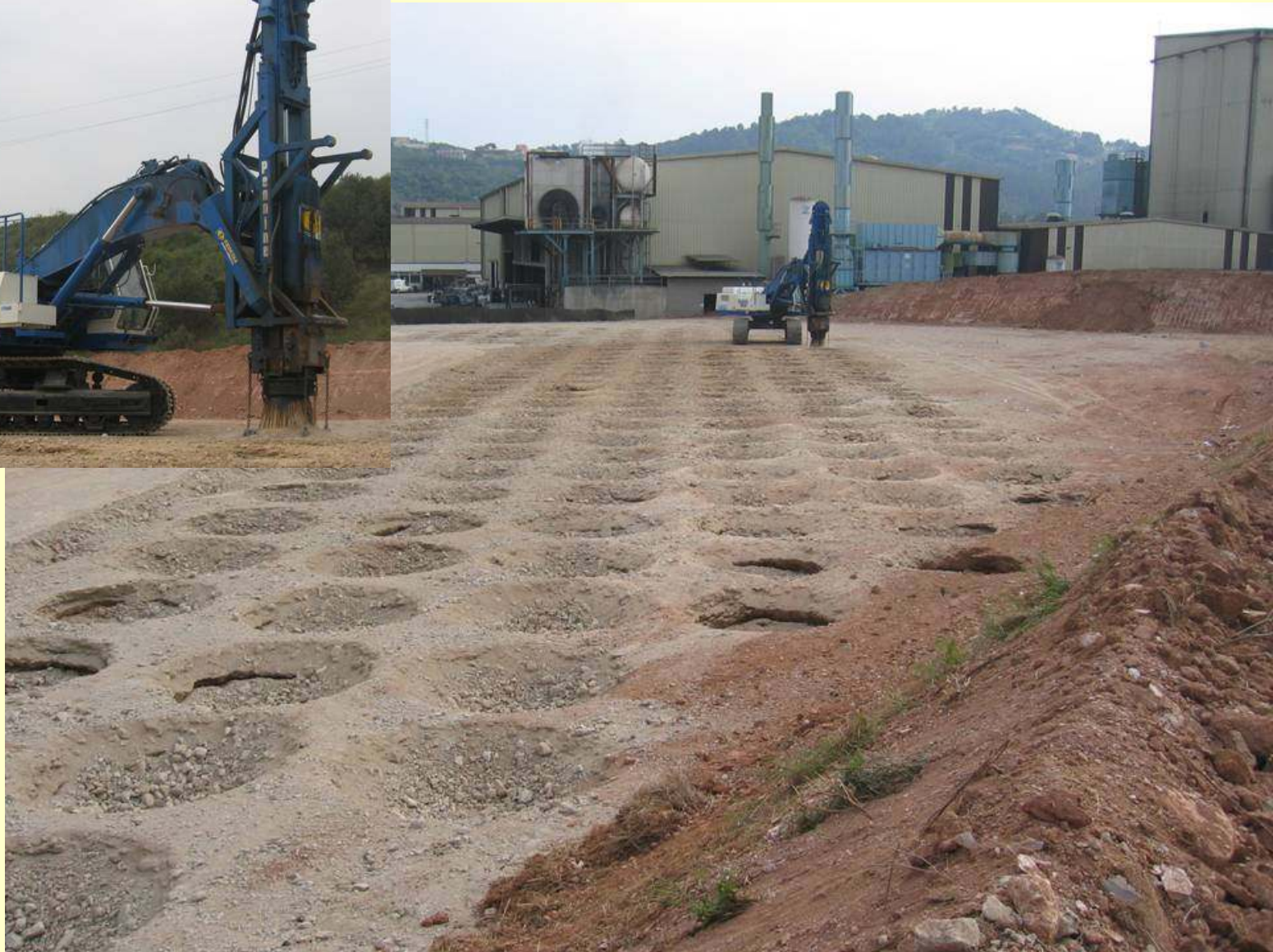
R apid I mpact C ompactor (RIC)
