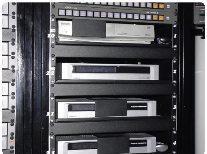
▲ The transmission signal is controlled with the help of standard HDTV receivers such as from Humax.
