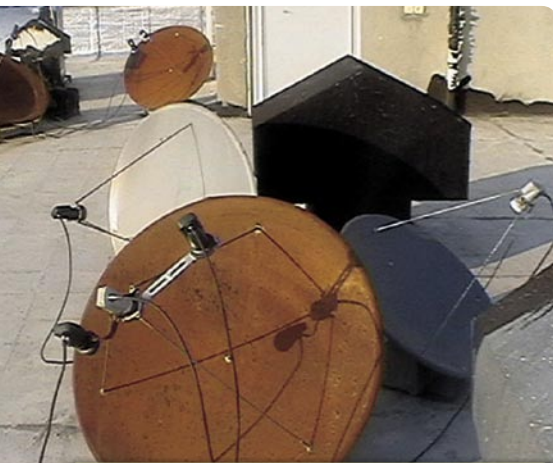
A flat roof has its advantages: plenty of space for the dishes. The dish in front even sports a home-made multifeed installation!
