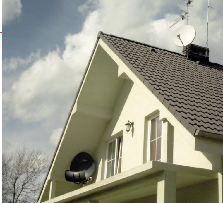
What do you prefer? A dish mounted to a motor on the top of roof, where it gets the full viewing range, or a fixed dish in some corner of your balcony to catch a smaller but sufficient range of satellites?
