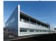
Customer Support and Training Center (Japan)
