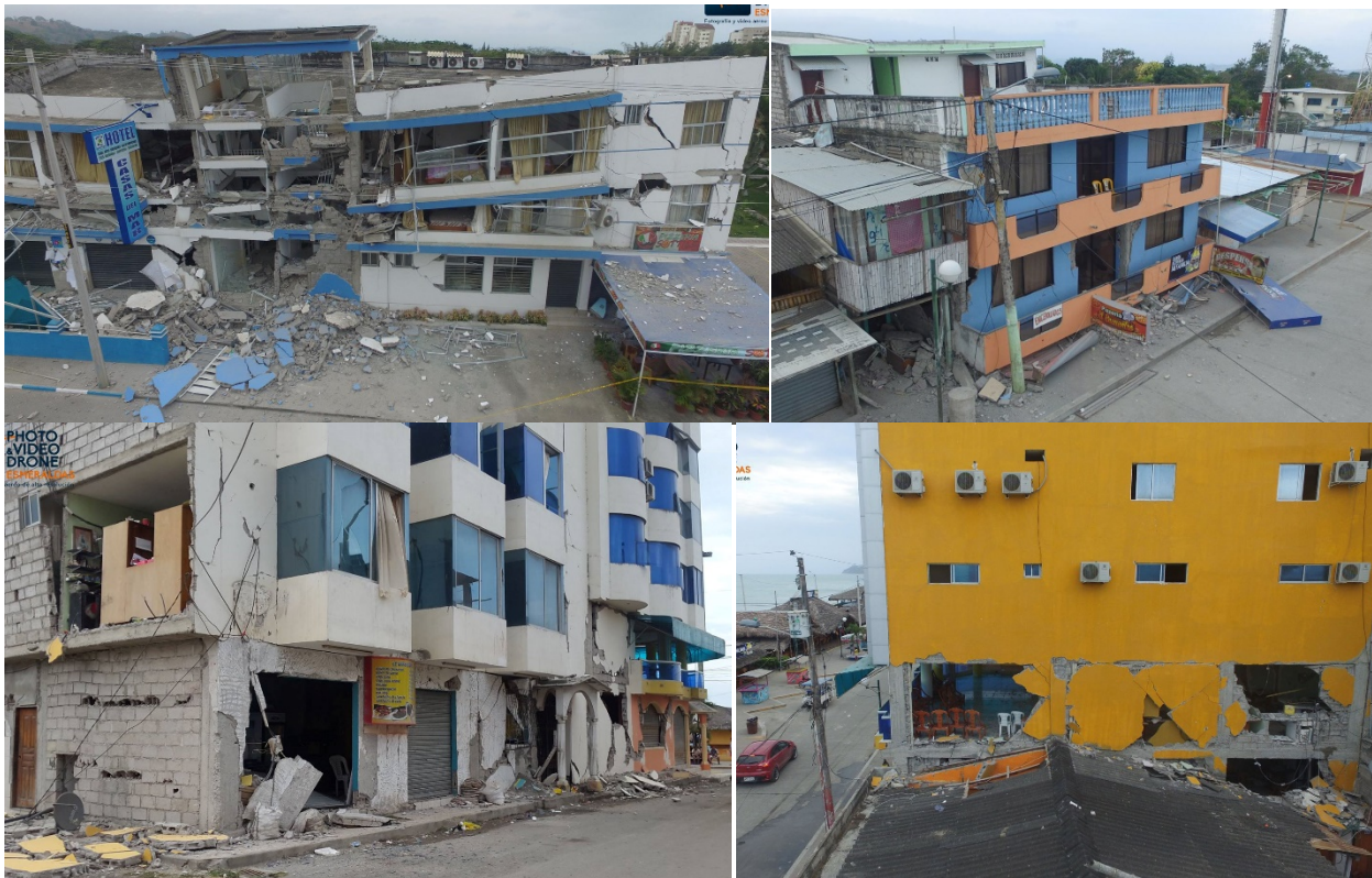
Figure 8a-d. Structural damage caused by the earthquake of 19 December 2016 (Mw 5.4, hypocenter 4 km). Upper images from left to right refer to the collapse of foundations at the Atacames site. Bottom images from left to right, referring to the site Tonsupa, province of Esmeraldas. Photo courtesy: "photo & video drone Esmeraldas".
