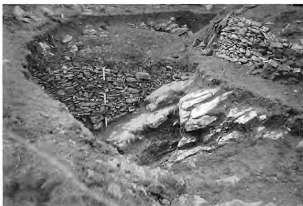
b Gorsey Bigbury. Ditch on West Side and Method of Excavation.
