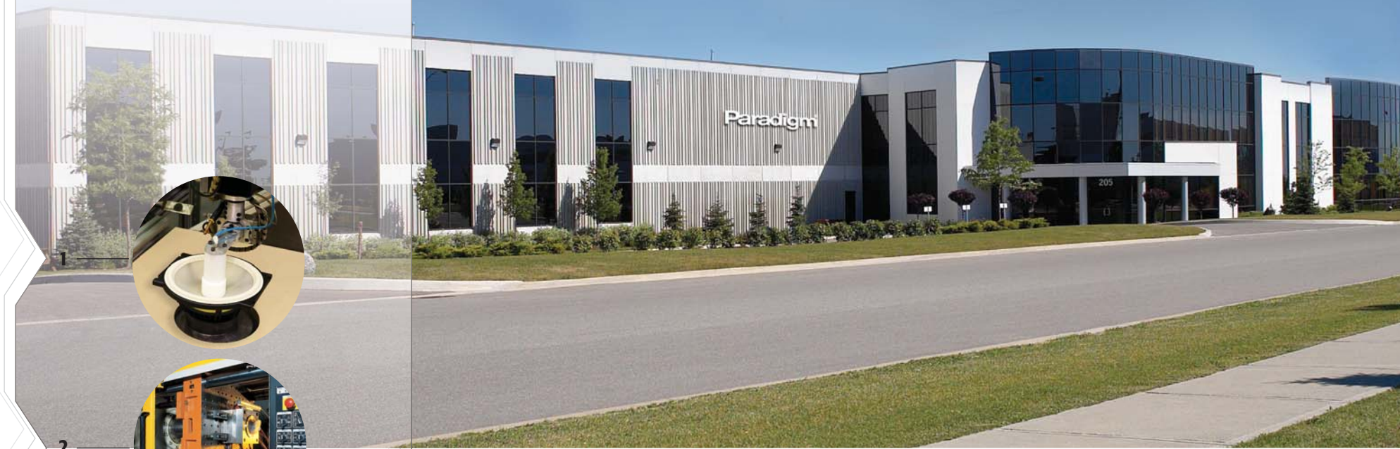
Paradigm's 225,000-sq.-ft. (21,000 sq. m) manufacturing facility and headquarters
