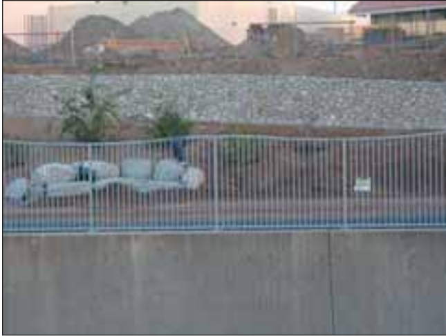
Figure 8.19 Decorative tubular steel fence along the Los Angeles River in Studio City
