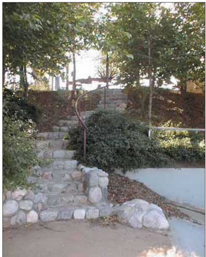
Figure 8.23 Stone steps with metal railing on the Los Angeles River at Rattlesnake Park
