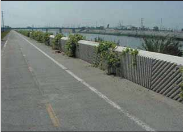
Figure 8.25 Concrete, textured parapet wall along the Los Angeles River in Long Beach
