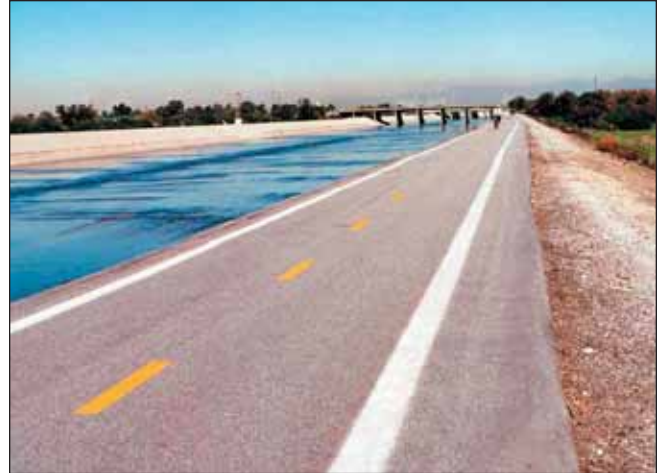
Figure 4.7 Leveed trapezoidal condition in Long Beach
