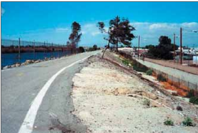
Figure 2.9 Previous conditions along the river in Long Beach
