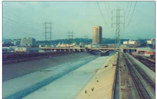
Figure 4.2 Entrenched trapezoidal condition at Fourth St. Bridge.
