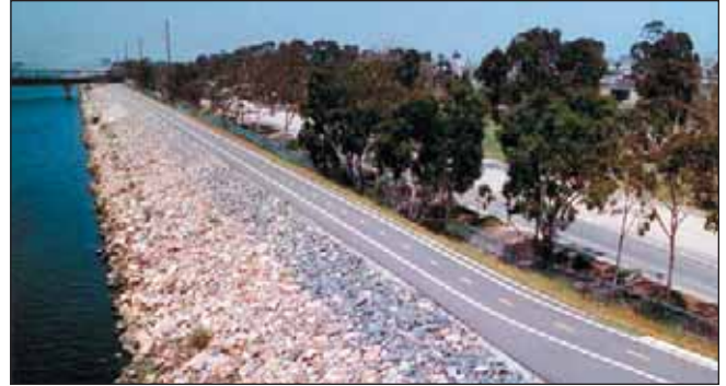
Figure 5.4 Los Angeles River Bike Path, no fencing on trapezoidal channel
