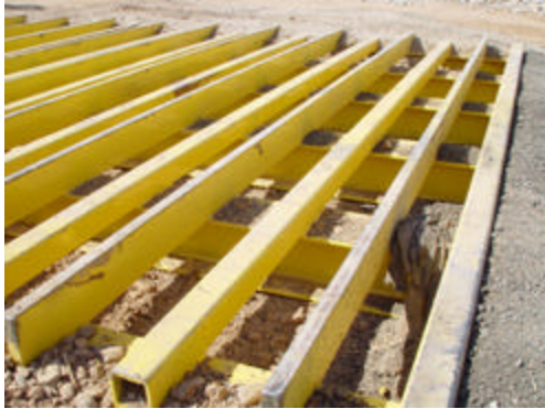
Figure 1: Grizzly rumble grate used to prevent track-out.
