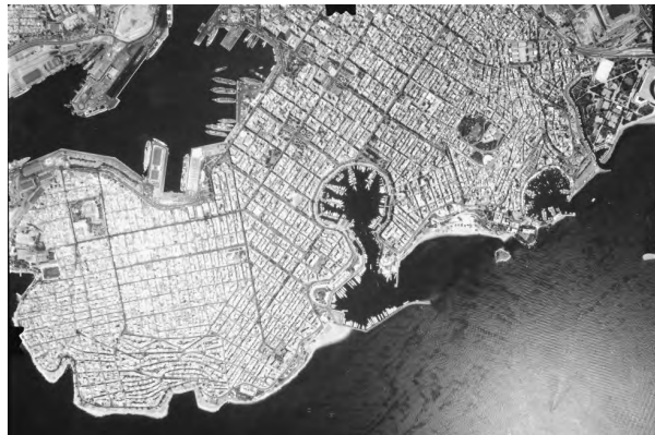
Figure VIII.2: Aerial photos showing the urbanisation and the anthropogenic uses along the coastline of the city of Peiraia (port of Peiraias, small yachting marinas, regulation of the Kifissos river outflow, sport constructions and changes of the coastline through deposition of earth material).
