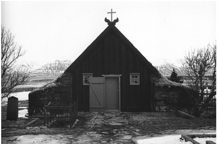
Víðimýrarkirkja, an Icelandic church built in the ancient manner of turf and stone
